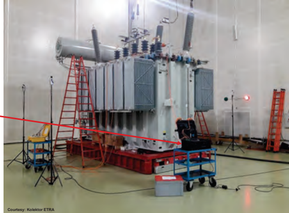
Transformer during Heat Run Test
